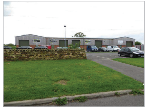
Timber cladding maintains a rural feel on an industrial building
