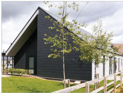
Artificial slate roofing and cladding fits a modern building into its context
