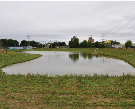
Photograph of completed retention pond in the southern field opposite Eden Camp.
