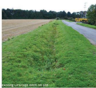
Existing Drainage ditch on site
